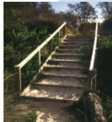
Figure 4.11b Timber steps provide access across foredune, protecting vegetation.
