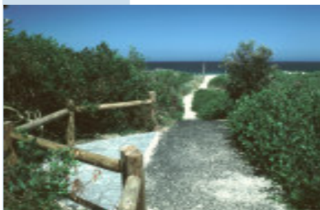
Figure 4.10e Asphalt provides access to a hind dune crest; bare sand extends to the beach.
