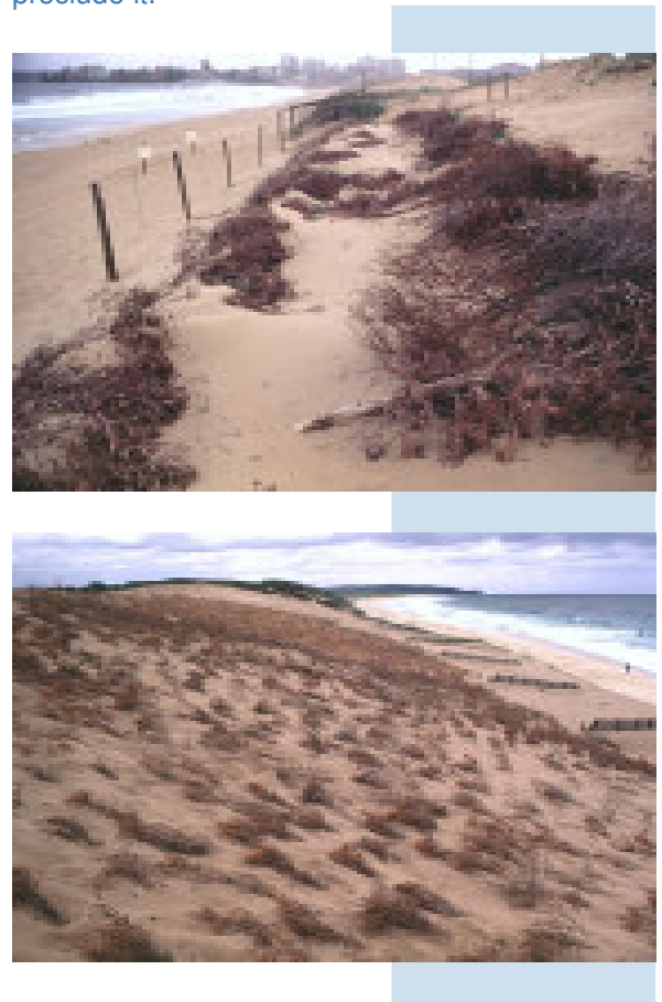
Figure 4.3 Brush matting is essential at exposed sites to protect bare sand until new plants are established.
