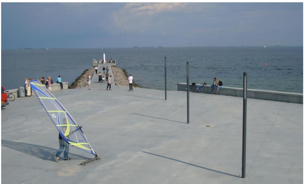
Figure 18.11 Amager Beach Park, Copenhagen, headland designed as recreational pier.
