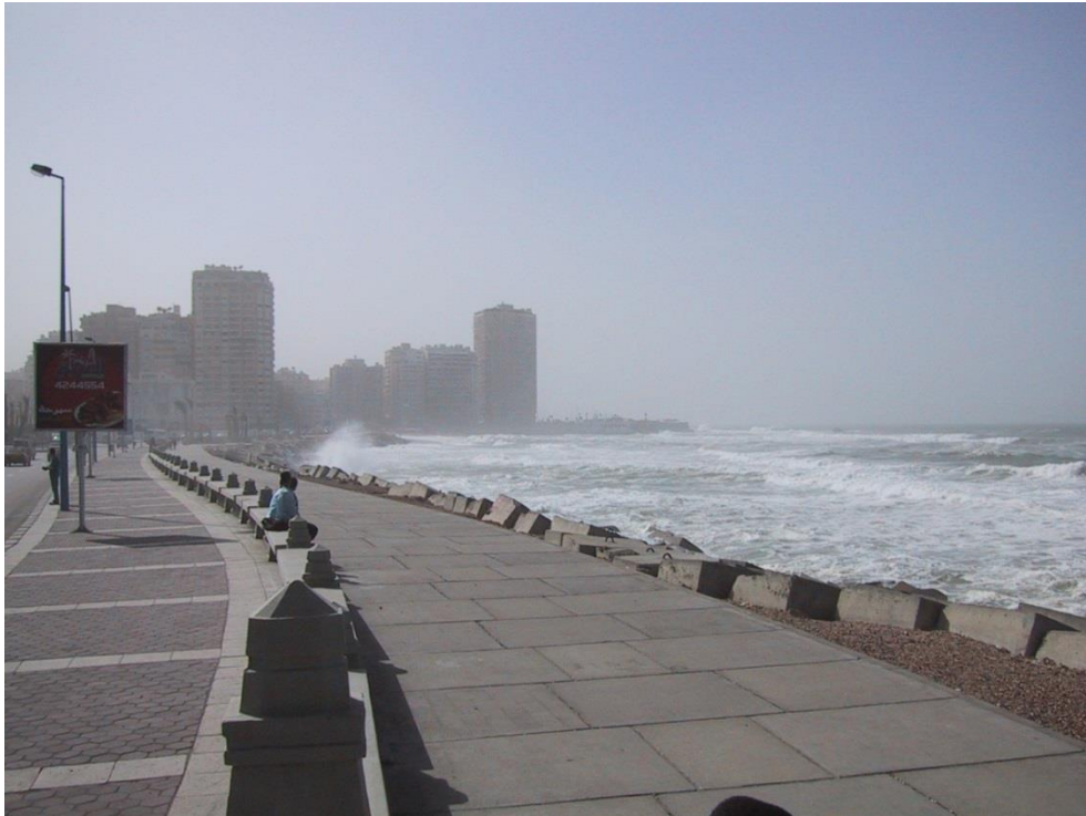
Figure 17.2 Seawall/revetment in front of Corniche in Alexandria.
