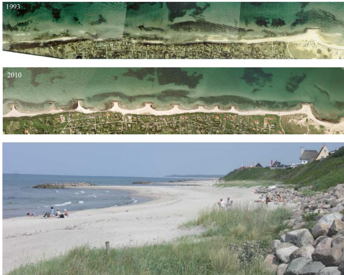
Figure 17.32 Breakwater protection scheme, Liseleje, Denmark. Upper panel: Situation before scheme. Middle panel: Aerial photo 12 years after construction in 1999. Lower panel: Situation in the middle of the scheme in June 2010. Project and photos by COWI. References: Helledie, C. (2011) and COWI (2012).
