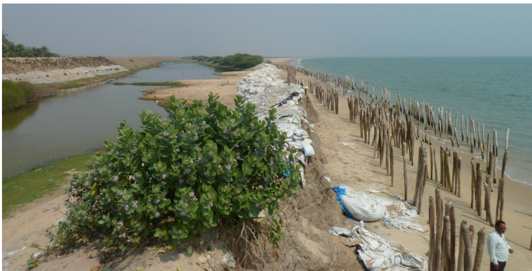
Figure 17.11 Emergency protection using grain bags and piles, Odissa, India.
