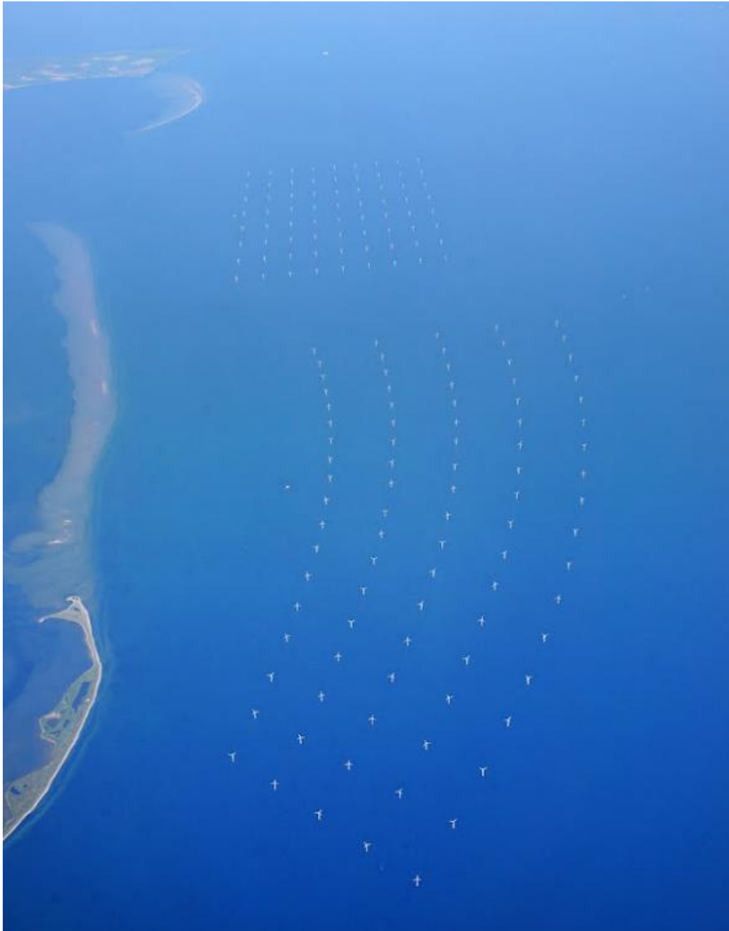
Figure 19.16 Rødsand I and II offshore wind power plants, off the Danish coast in Fehmarnbelt, Denmark. © Pavlo Dyban.
