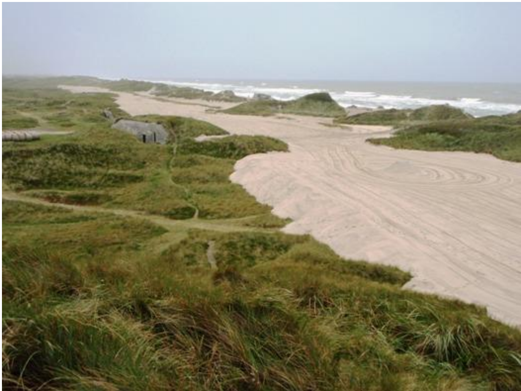
Figure 17.59 Dune reinforcement by widening the dune landwards from the landwards slope of the existing dune, from the Danish North Sea Coast.
