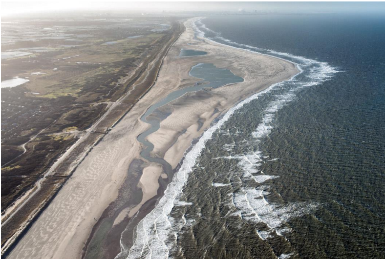
Figure 17.51 The development of the Zandmotor mega nourishment. © Zandmotor.
