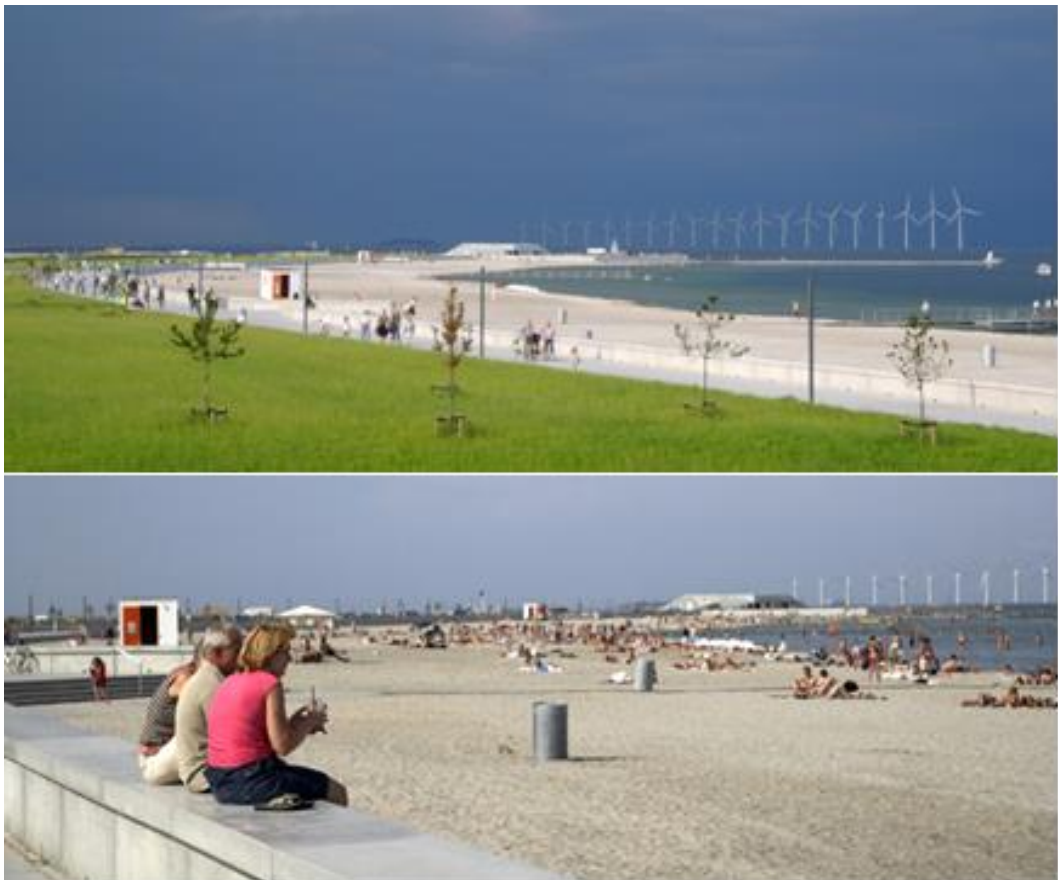
Figure 18.18 Amager Beach Park, Copenhagen. Upper: Promenade separated from the beach by a seawall. Lower: Seawall along the southern beach section having multiple functions: Coast protection, separation between promenade and beach and sitting furniture.
