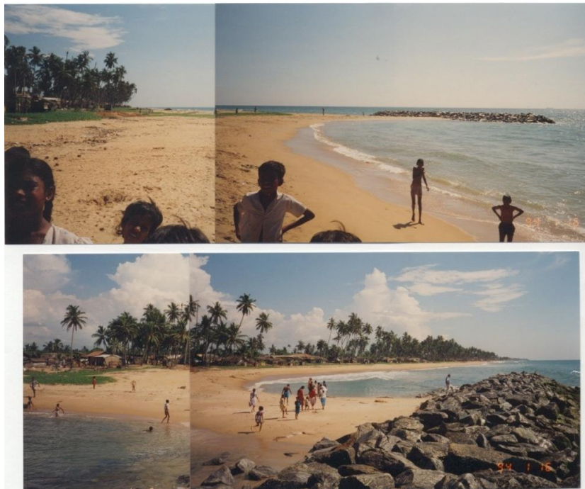
Figure 17.28 Coastal breakwater, which has formed (an unstable) tombolo, Covis Place, Sri Lanka. L_B^* = 0.8, X^* = 1.0 .
