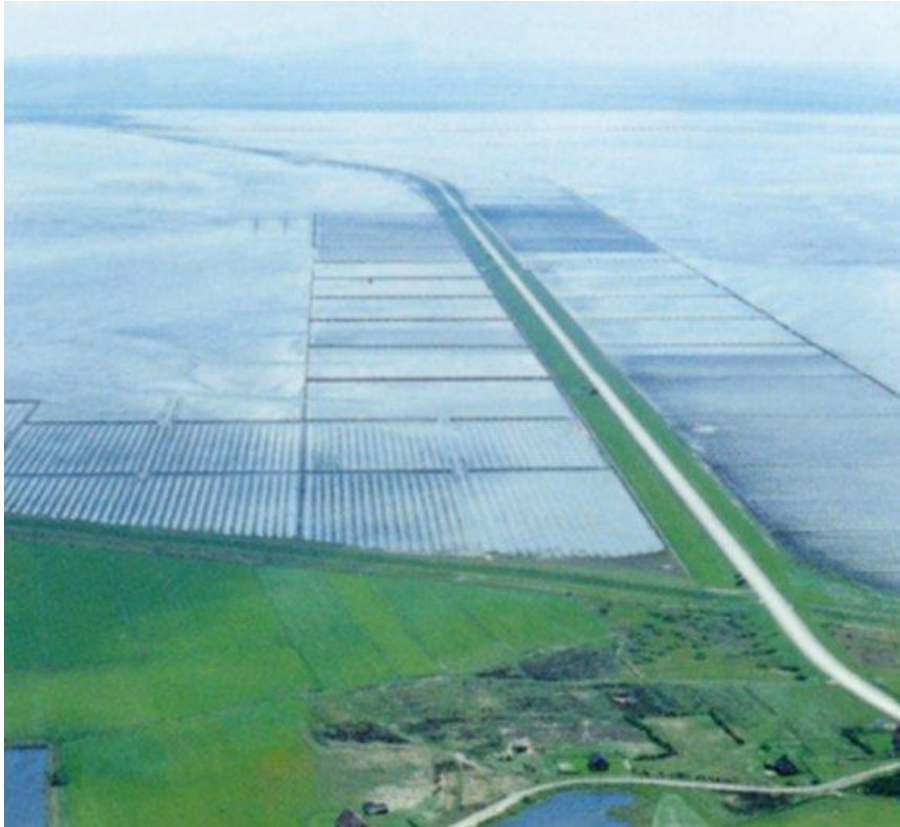
Figure 17.62 Siltation traps for the enhancement of natural platform growth.
