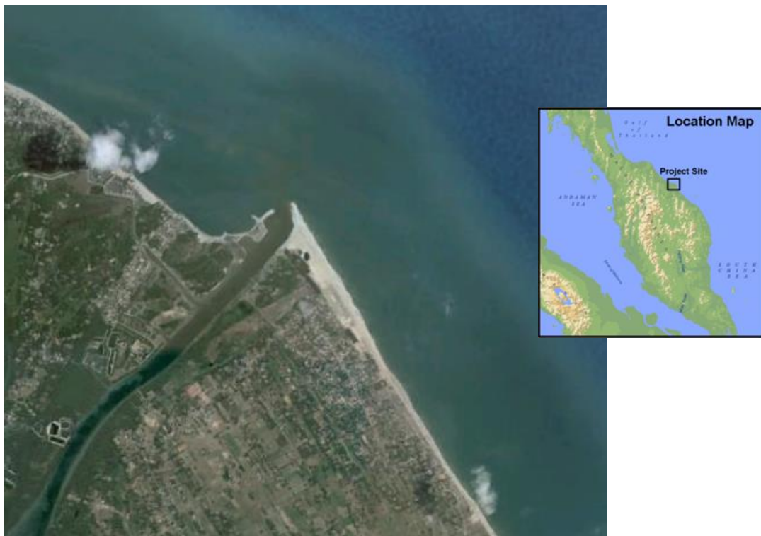
Figure 4.2 Example of accretion and erosion in delta area upstream/downstream, respectively, of Pengkalan Datu river mouth regulation works, Terengganu State, Malaysia.
