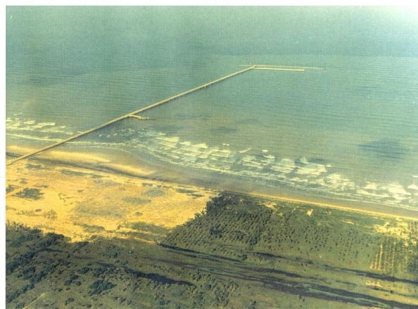
Figure 17.27 Sand accumulation forming a salient in the shoreline behind an offshore breakwater, Sergipe, Brazil. L_B^* = 0.22 , X^* = 3.6 .
