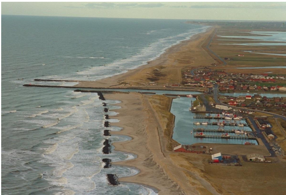
Figure 19.5 Aerial photo of Thorsminde Tidal Inlet (before re-design) on the North Sea Coast of Denmark. The fishing port is an attachment to the channel on the seaside of the sluice; Part of Nissum Lagoon can be seen to the right.
