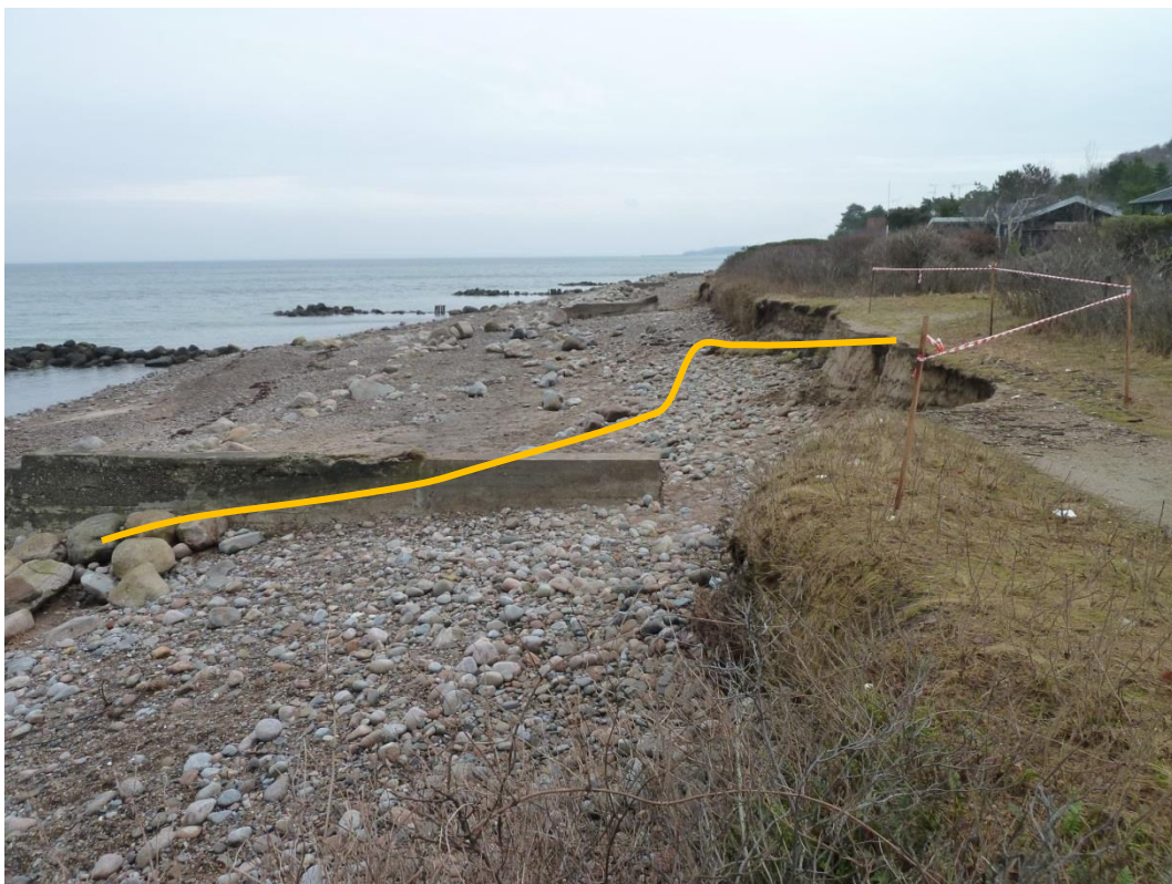
Figure 17.24 Acute erosion of beach and cliff despite groyne protection. Villingebæk, North Sealand, Denmark following the extreme storm “Bodil” on 6 th December 2013. Yellow line indicates estimated beach profile before storm.
