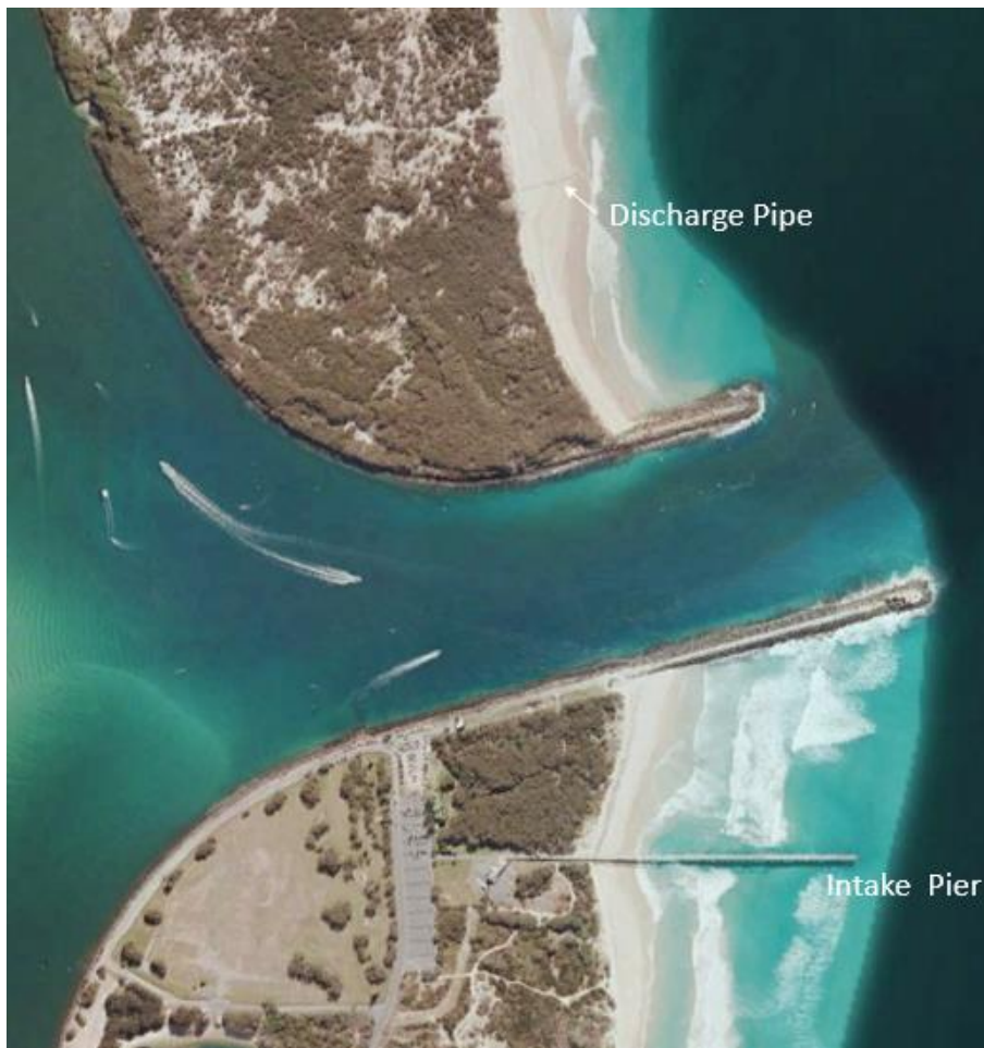
Figure 19.12 Gold Coast Seaways, Australia. Bypass arrangement. (Google Earth).
