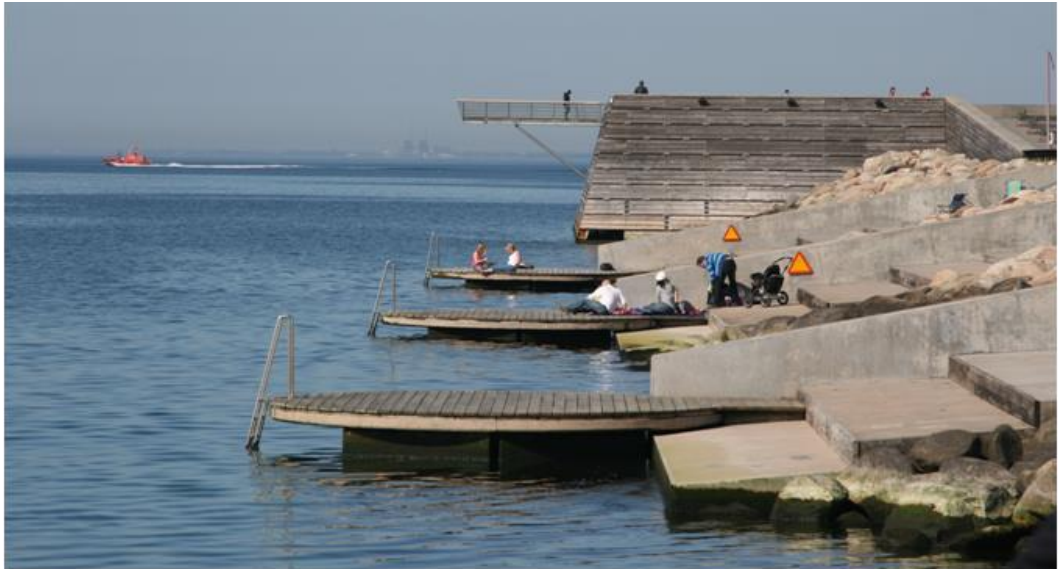
Figure 18.17 Malmø West Harbour, revetment equipped with steps and platforms for access to the water.
