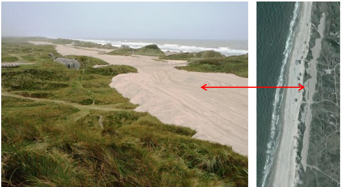
Figure 17.49 Dune nourishment at Kryle at the Danish North Sea Coast. Left: photo; Right: satellite image.
