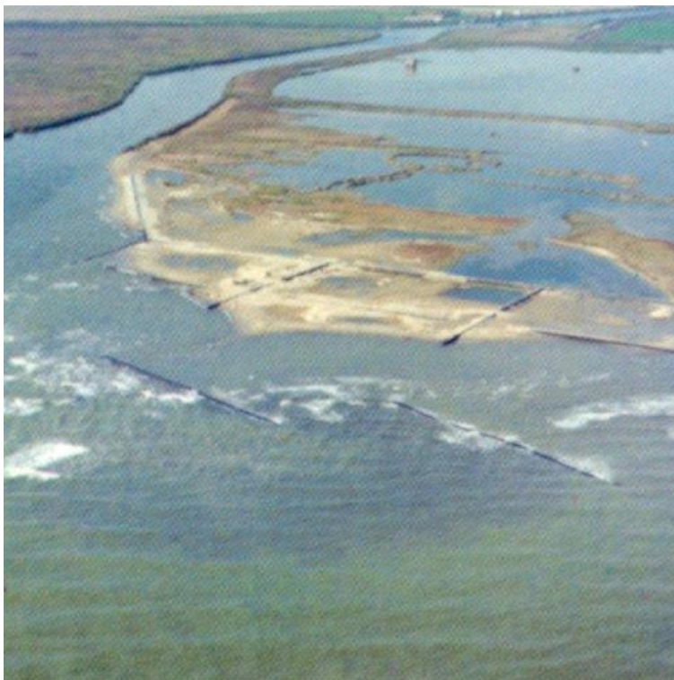
Figure 17.36 An example of a protection scheme at the mouth of the Po River, Italy, consisting of bulkheads and submerged breakwaters (photo taken at low tide).
