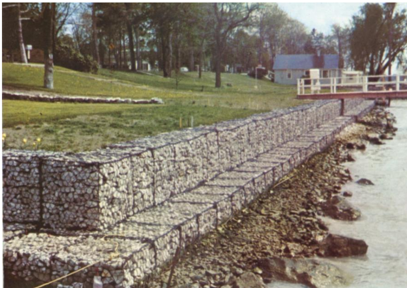
Figure 17.15 Example of bulkhead structure constructed by Gabion mesh boxes.
