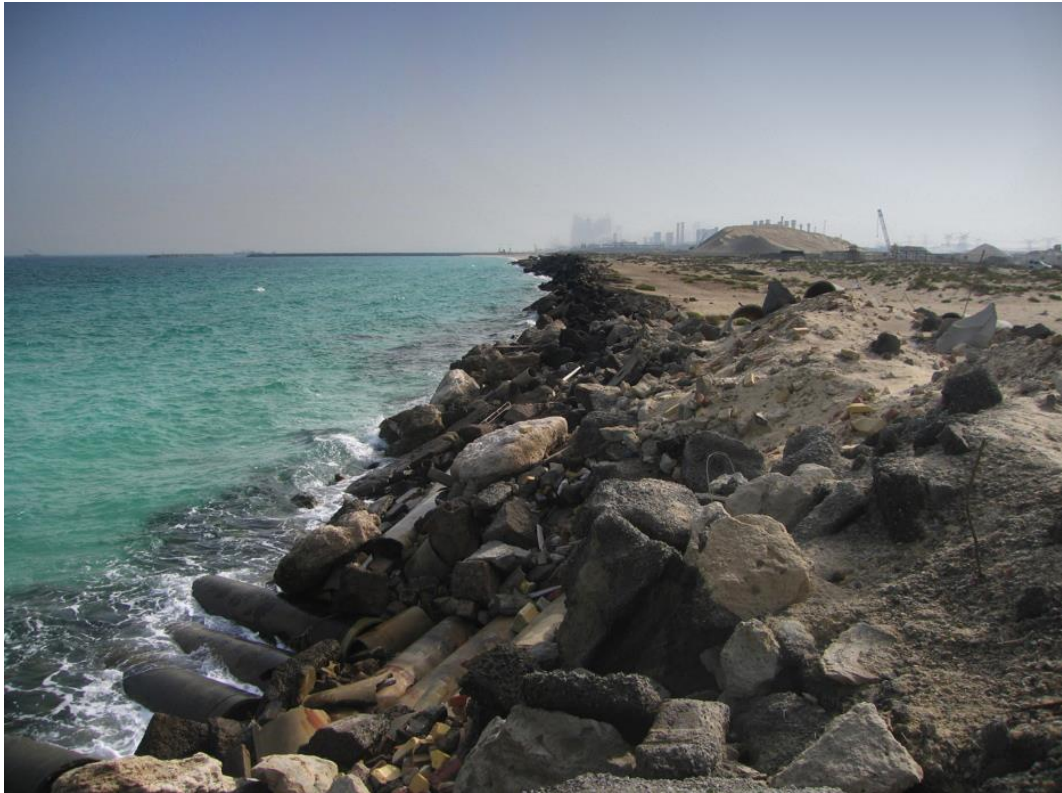
Figure 17.14 Emergency revetment constructed by concrete rubble, Dubai.
