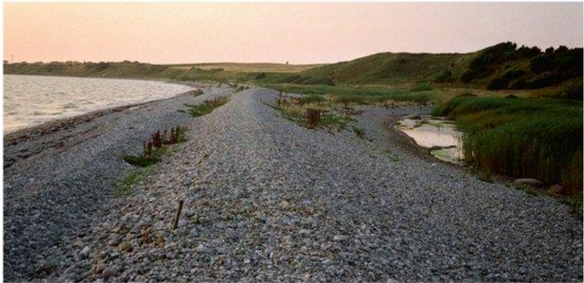
Figure 17.47 Shingle beach with beach berm forming natural defence of low-lying hinterland.
