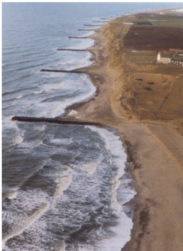
Figure 17.17 An old groyne field protection at the Danish North Sea Coast, constructed in concrete blocks.
