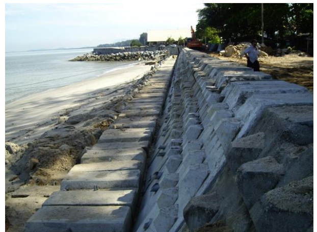
Figure 17.7 Sketch of concrete block revetment (Labuan blocks) (left) and photo of installed units (right).
