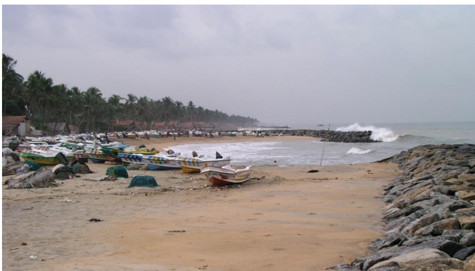
Figure 17.41 Layout of a cove (upper) and photo of a cove (lower) constructed at the SW coast of Sri Lanka.
