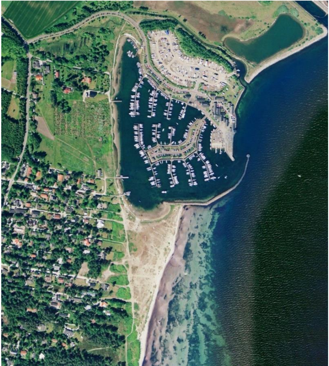
Figure 18.12 Kalø Vig Marina, Denmark. Marina with detached breakwater providing soft transition between beach and marina.
