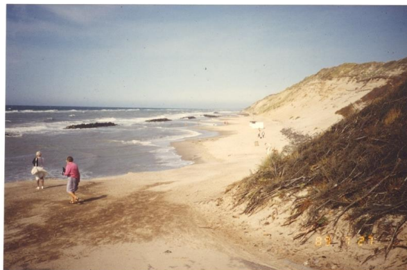
Figure 17.29 Beach breakwaters, The Danish West Coast. L_B^* = 1.0 , X^* = 0.14 .
