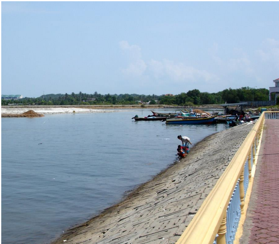
Figure 17.6 Flex Slab revetment along river bank, Labuan, Malaysia.
