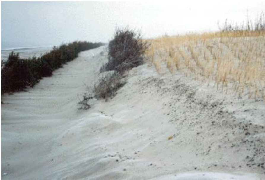
Figure 17.43 Marram planting and the placing of spruce fascines in wind alleys (Danish Coastal Authority).
