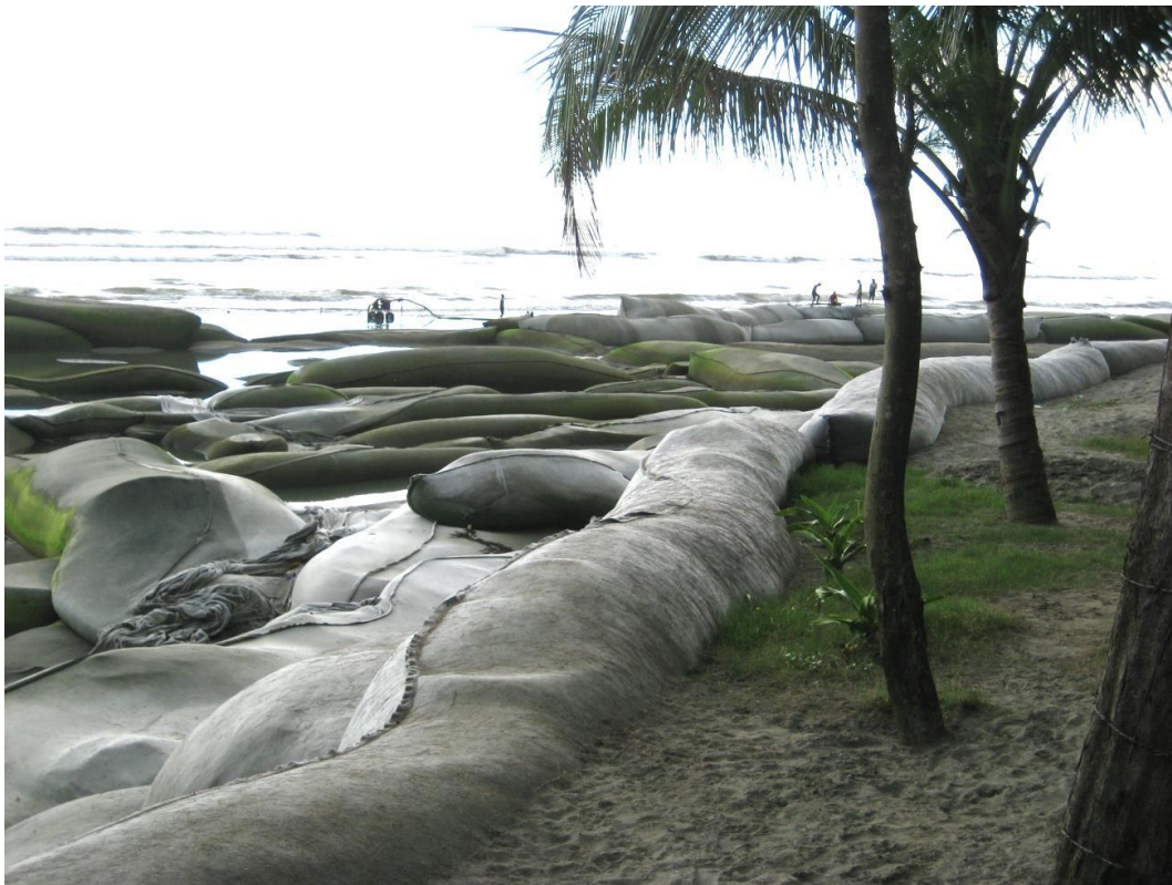
Figure 17.10 Revetment constructed by geotextile sand tubes, note partly collapsed tubes and unnatural appearance. Marine Drive, Cox's Basar, Bangladesh.
